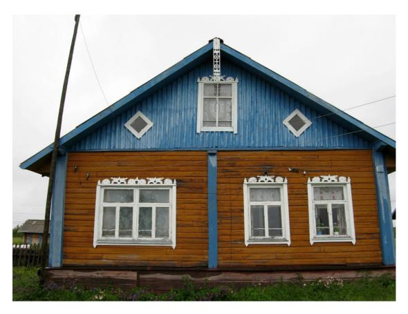
Figure 8: A nineteenth-century house in Jyskyjärvi village, Russian Karelia. It illustrates how a light timber structure, lacking ground-set foundations, can be well-finished and decorative, with architectural pretensions. Like the hall-type buildings on post-Roman sites in northern and western Britain, its archaeological traces would be fugitive. (Photograph John Blair.)
